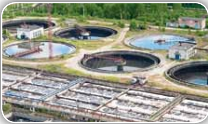
WATER AND EFFLUENT TREATMENT
