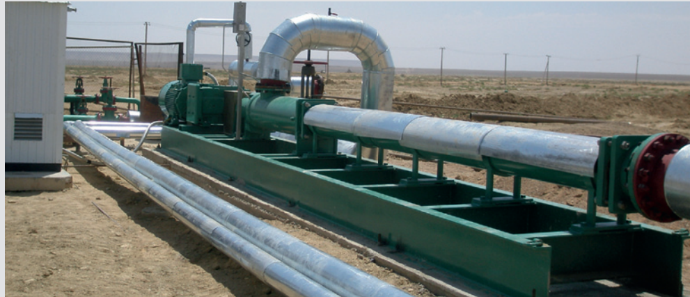
Adapting to the occasional challenges: The final pipeline lagging read for a cold winter in a remote Kazakhstan. Commissioning teams are always on hand to help up and cure unforeseen start up challenges.
