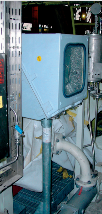
Instrumentation located in a heated cabinet
