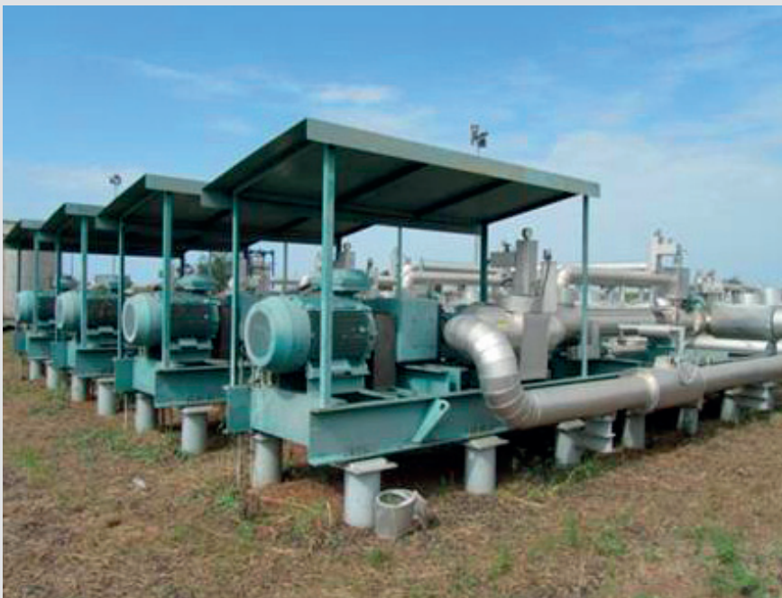
NETZSCH service team condition monitoring survey photo
