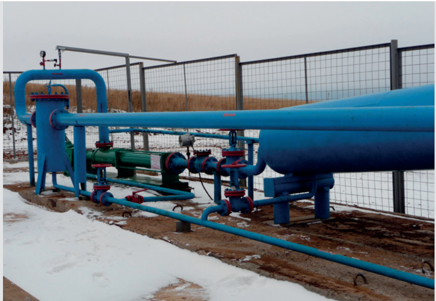
NETZSCH pump operating in remote Russian multiphase crude oil application, with liquid collection
