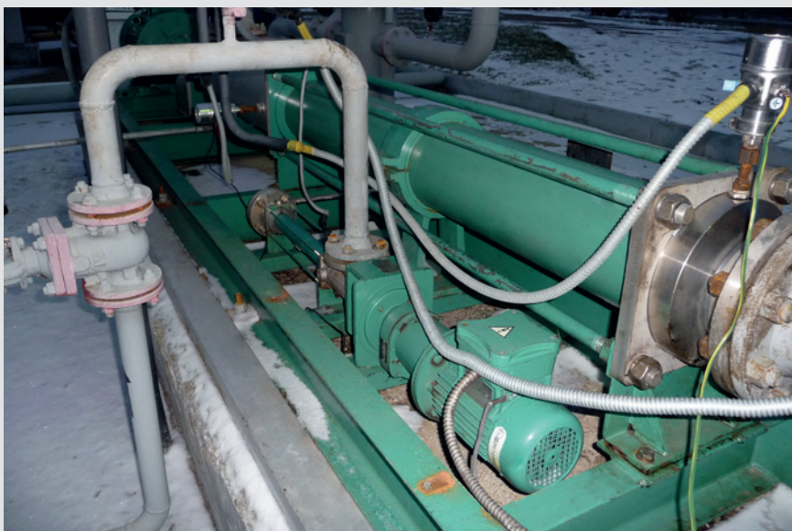
NETZSCH pump operating with 85% GVF at oilfield in Russia. Small injection pump for lubrication working when GVF is high.
