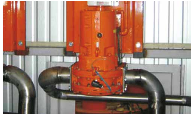
Vertical TORNADO® pumps to transfer lubricating oil on board
