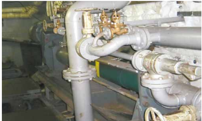
NEMO® pump, to transfer drilling mud
