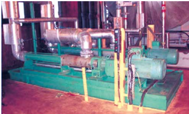
NEMO® pumps on platform to transfer drilling cuttings and sludge
