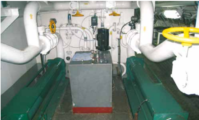
NEMO® pumps, to transfer kaolin on board
