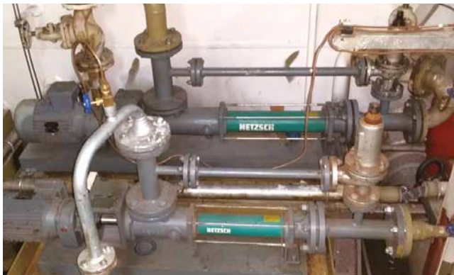
PC pumps in engine room
