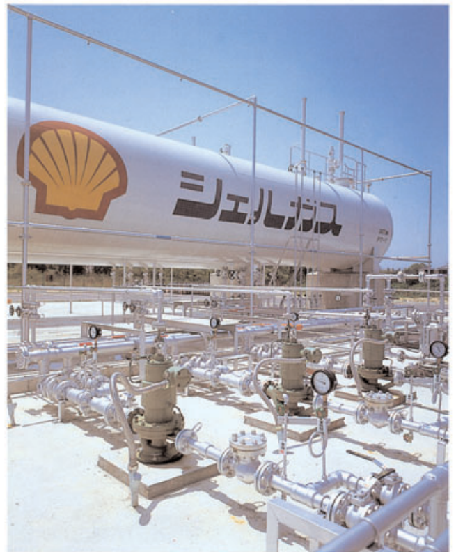
LPG Transfer in LPG Filling station (Vertical In-Line Type, Reverse Circulation)
