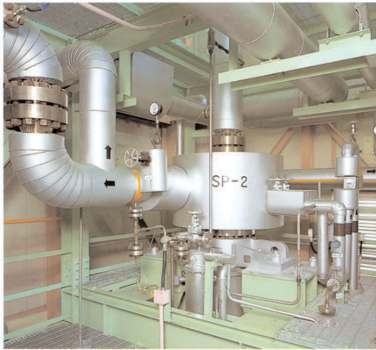
High Temperature & High Line-Pressure Service in Nuclear Power Station
