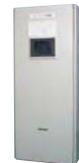
Water conditioning control panel
