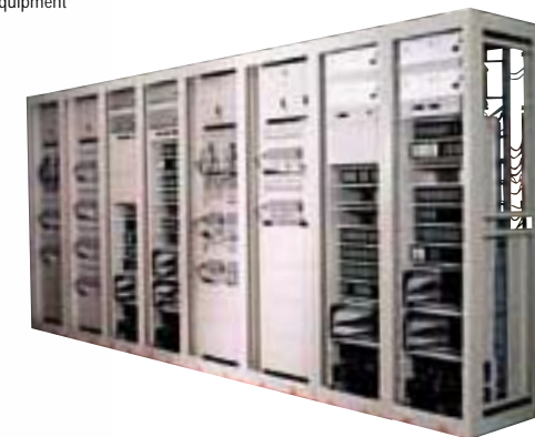
Automatic boiler control system
