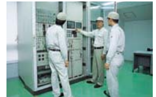
Training of instrumentation & power systems
