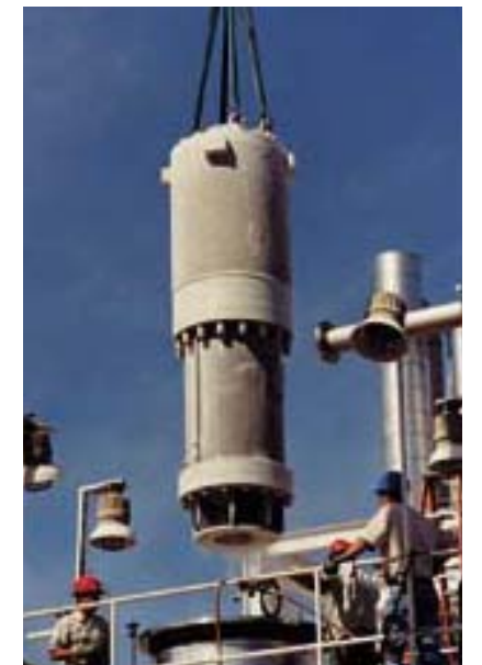
Cryogenic Pump ( Submerged wet motor type pumps for liquefied gases )
