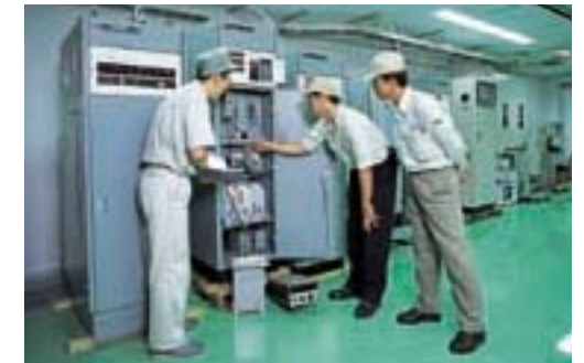
Training of instrumentation & power systems
