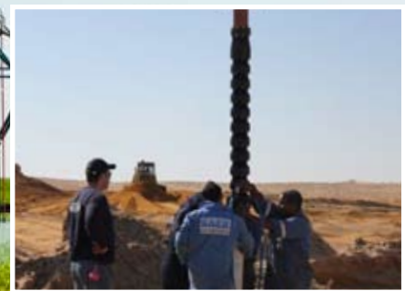
Submersible deep well pump being installed in Egypt.
