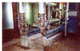
Crystallization seepex pumps BN 17-24, product: molasses, flow: 15 m 3 /h / 66 usgpm, speed: 360 rpm, pressure: 12 bar / 170 psig, temperature: 55° C / 131° F, viscosity: 7000 mPas, SG: 1.4 kg/dm 3
