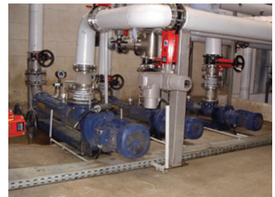
seepex BN range pumps for transport of manure / fat mixture
