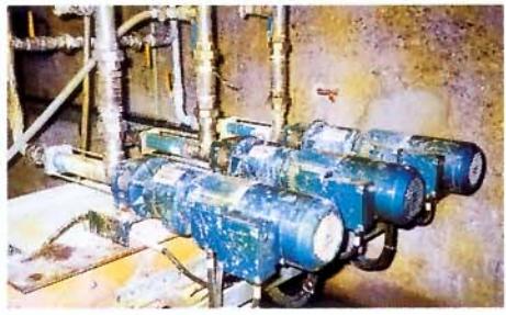
(aluminium hydroxide chloride sulphate), flow rate: 10 - 300 l/h, speed: 15 - 180 rpm, pressure: 4 bar (60 psi), temperature: 20 - 30° C, spec. gravity: 1.2, pH-value: 1 - 7, viscosity: 20 - 80 cps
