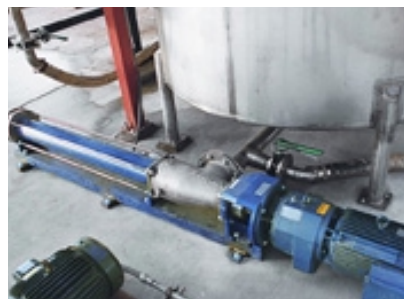
seepex pump BN 5-24, Product: sediment, Pressure: 4-6 bar (60-90 psi), Capacity: 2m 3 /h (8.8gpm)
