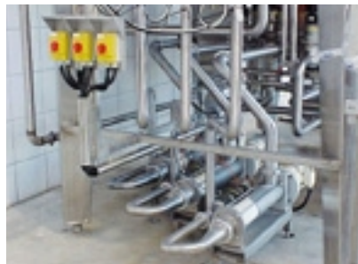
seepex pumps BCSB 52-6L Product: cream, Pressure: 4 bar (60 psi), Temperature: 5-20°C (40°-70°F), Capacity: 10-40m 3 /h (44-176gpm)
