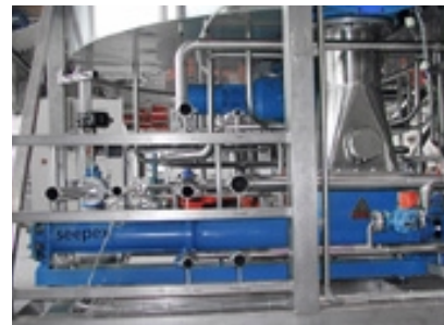
seepex pump BT 17-12 , Product: spent grain from clarification tub to further processing as animal feed, Pressure: 4 to 10 bar (60-150 psi), Viscosity: up to 15,000 cPs, Temperature: 70-80°C (160-175°F), Capacity: 8m 3 /h (35.2gpm)
