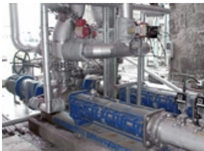
seepex pumps BN 130-12, Product: distillery mash, 10%DS, Viscosity: 2000 cPs, Temperature: 65°C (150°F), Pressure: 8-12 bar (120-175 psi), Capacity: 40m 3 /h (175gpm)
