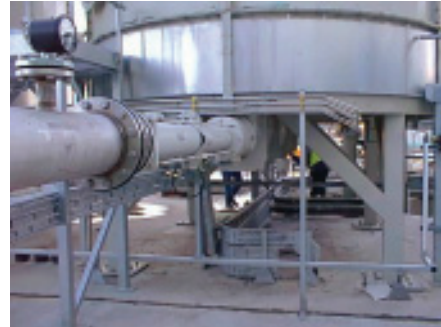
seepex silo discharge pump mounted below a silo for conveying dewatered sludge
