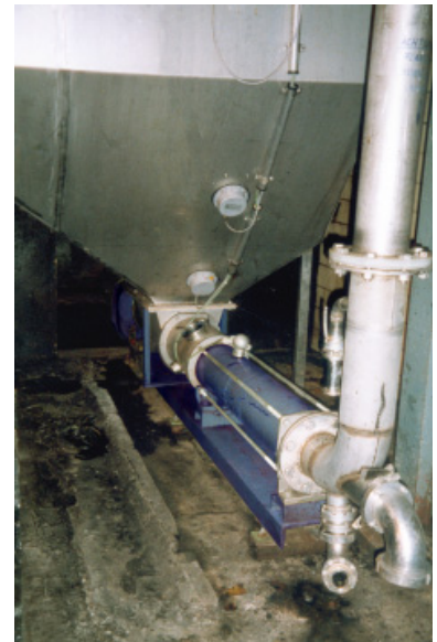
seepex BTM range pump under storage container
