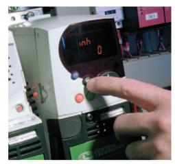
SM-Keypad, designed for use with Unidrive D, has two rows of 7 segment LED displays. These are very easy to see at distance and in poor lighting conditions. The upper display shows the drive status or the current menu and parameter number. The lower display shows the parameter value or the specific trip type.
